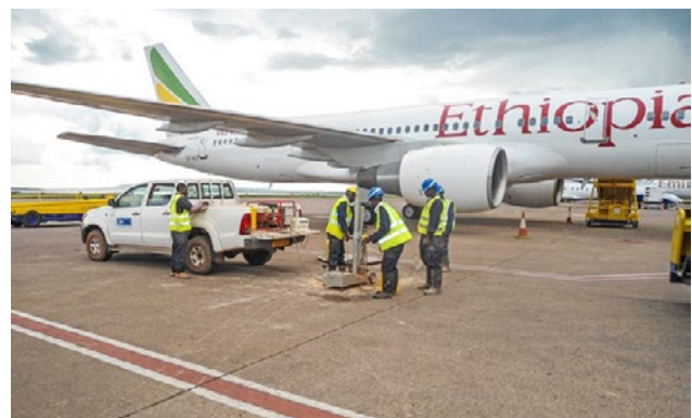
Pavement analysis at Entebbe Airport
